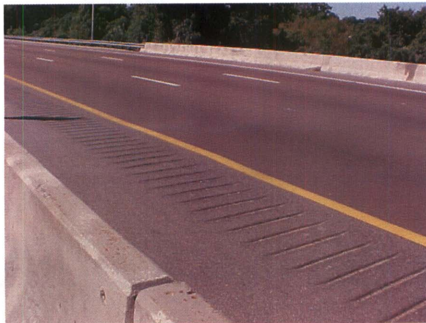
VIEW ACROSS TOP OF DECK, LEFT LANE
