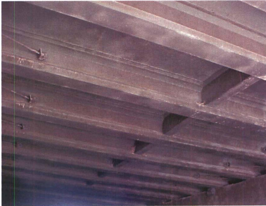
SPAN #2, BOTTOM OF DECK
