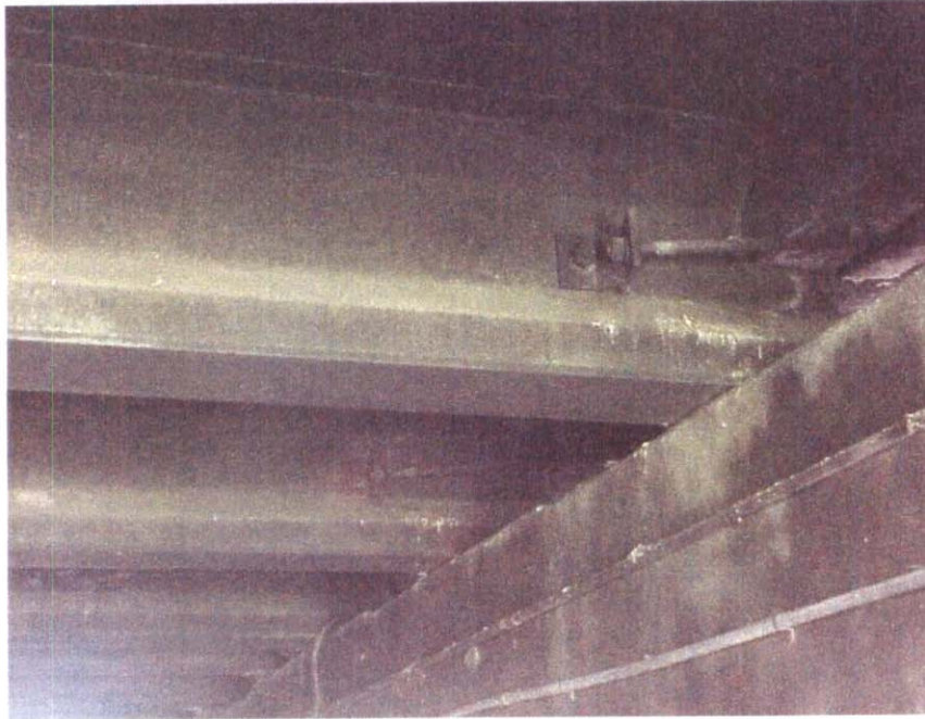
SPAN #3, SHOWING EARTHQUAKE DEVICES
