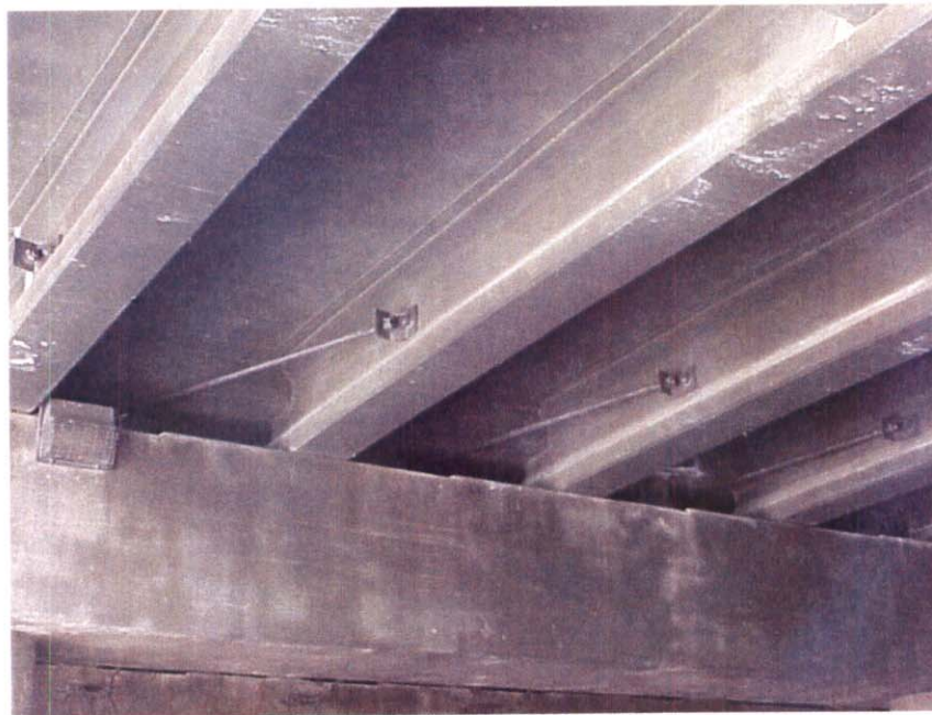
SPAN #2, SHOWING EARTHQUAKE DEVICES
