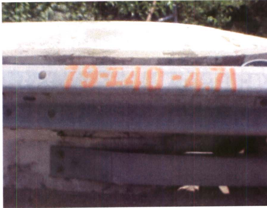
BRIDGE NO. ON RIGHT RAIL
