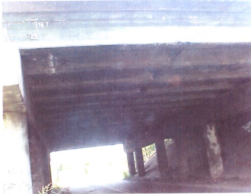
SPAN #2, BOTTOM OF DECK
